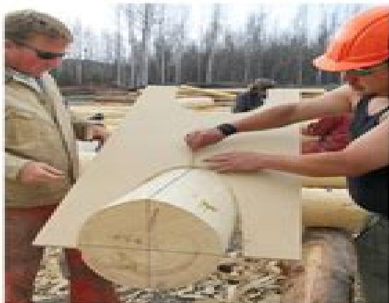
Figure 24: Dan and Hilo work on a truss in one of my hands-on courses. Note how the nail in hinge point helps position the flat surface that is used to trace the cut line onto the log. (This is sort of a portable C-jig, turned on its side.)
