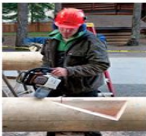
Figure 27: Left: Jordan chainsaws a tie beam joint where the rafter tail will be placed.
