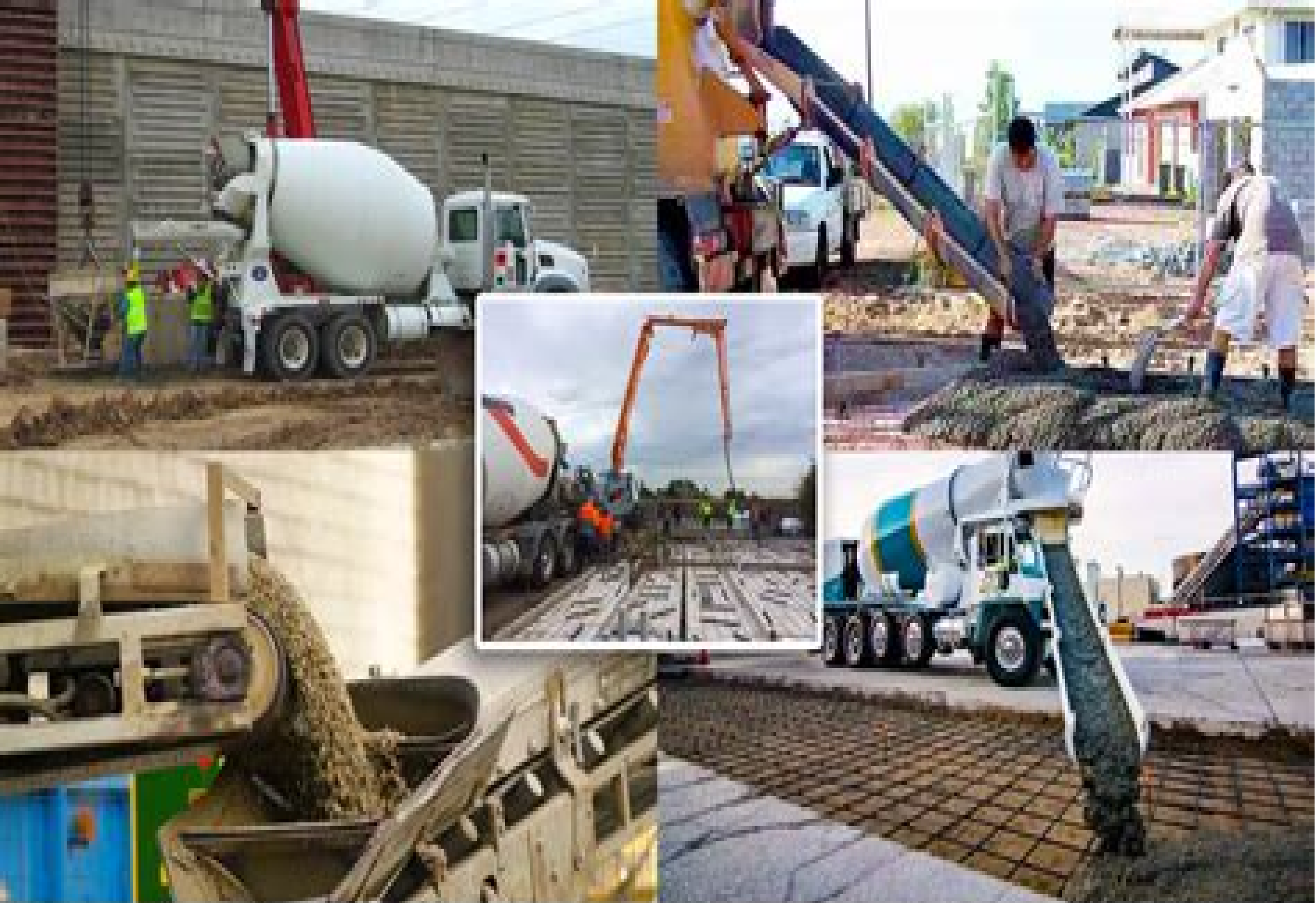
Effective Methods for Transporting and Placing Concrete
